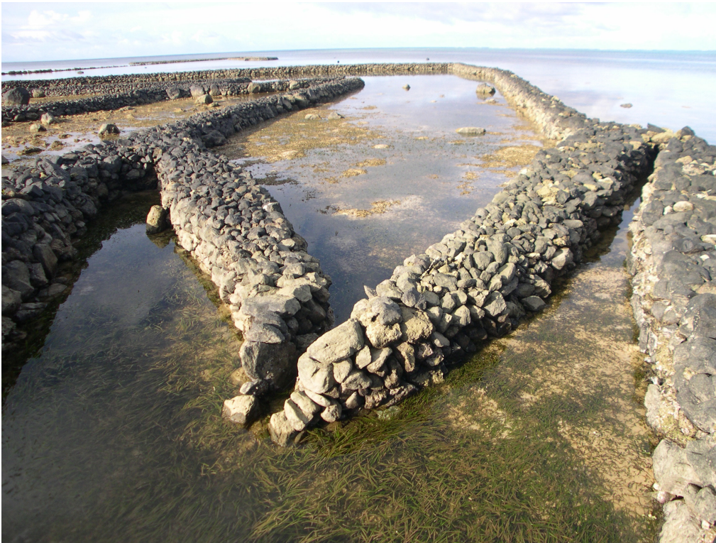
An aech, or fish weir, named “Daqoloch” in Rikeen, Yap. When tides are high, fishes swim into the structures. After the tide ebbs, they are trapped, either for immediate harvest or further cultivation. Fish weirs are found throughout the world and vary in size, material, and design. This aech is part of a larger collection throughout Yap. They are an important food source, profound source of cultural pride, and link ancestral practice to contemporary culture. Image courtesy of Bill Jeffery.
