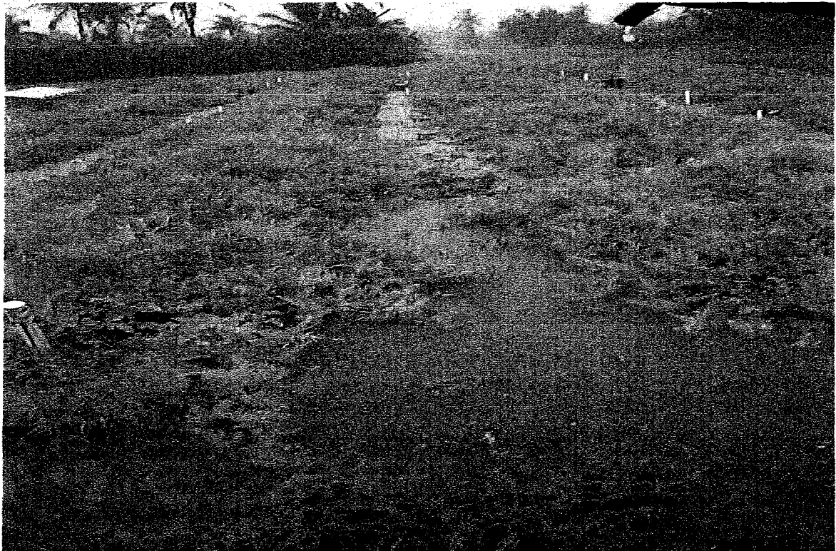
Picture 1: Field flooding from June 22 heavy rainfall event. Rain water began to laterally infiltrate the black plastic mulch on June 16 th leading to deep seepage and leaching.
