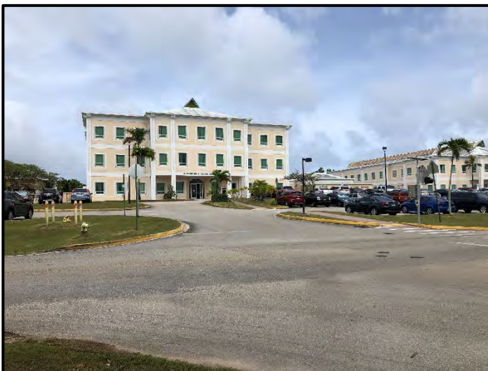
Photograph 9. The UOG campus was located across University Avenue, to the southeast of the subject property (15 March 2019).
