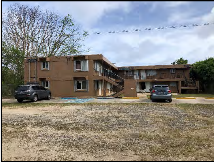
Photograph 4. One of the three apartment buildings located on the adjoining property to the south. This building was located along Atbut Lane to the south (15 March 2019).
